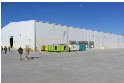
The construction project included four warehouses, like the one above, and an administration building. (Courtesy of the Special Inspector General for Afghanistan Reconstruction)
